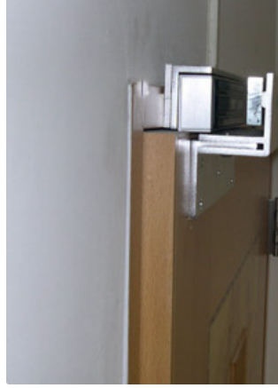
Installation of the Armature for Electromagnetic Lock
