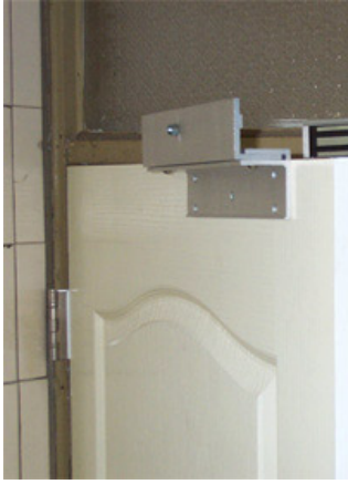
Installation of the Armature for Electromagnetic Lock
