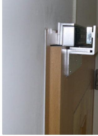
Installation of the Armature for Electromagnetic Lock
