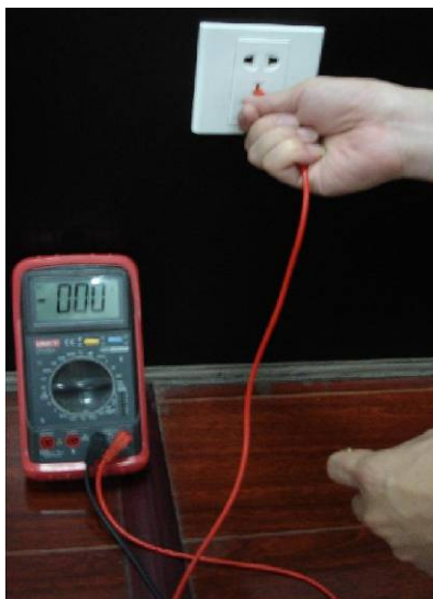
Appendix Figure 7-5 Check earth cable connection
